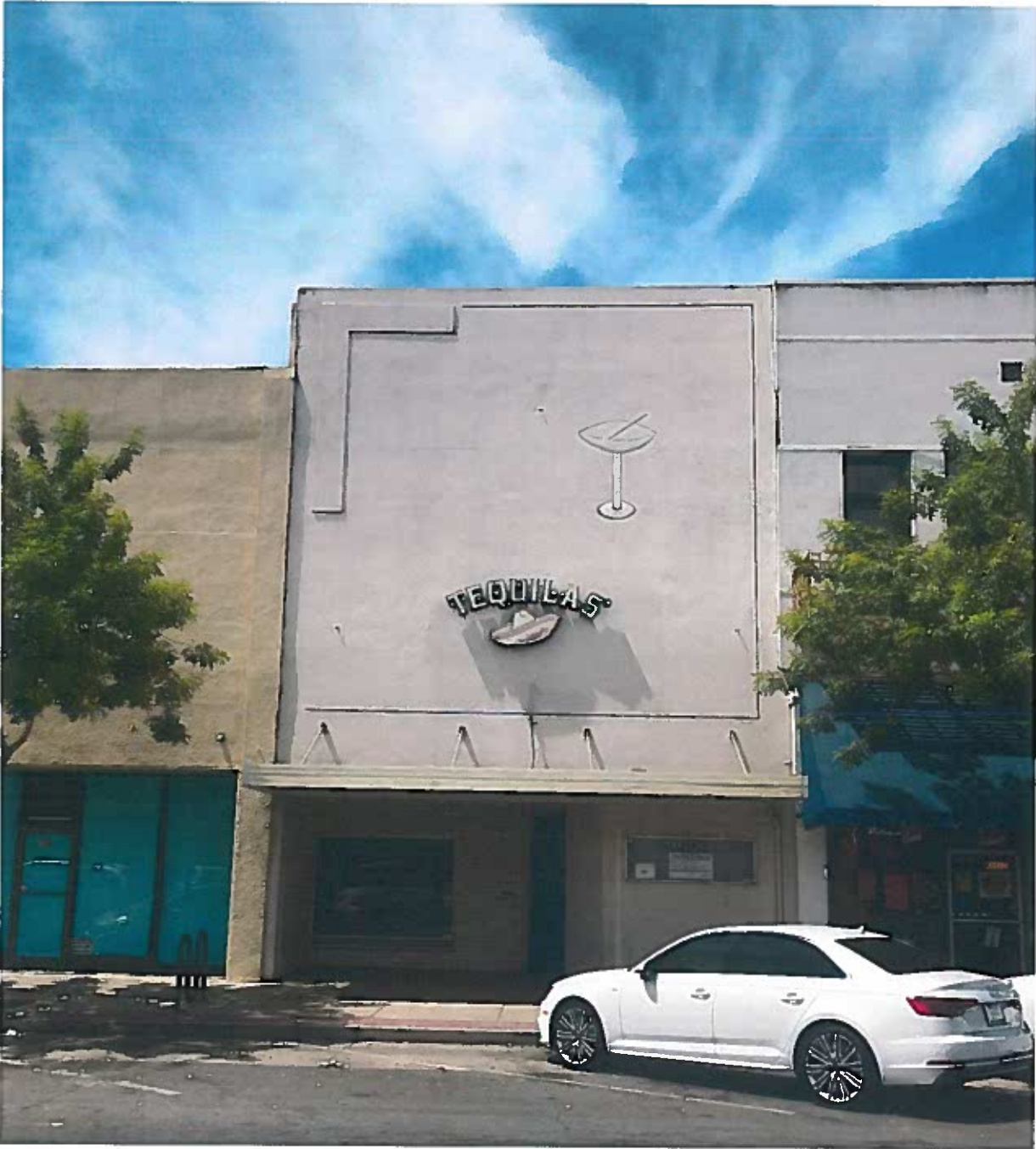
Seventh Street Facade
